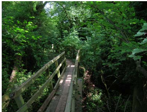
Footbridge over Bottom Dumble
